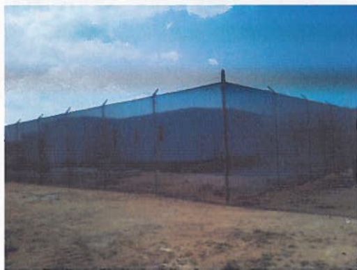
Security Fence installation in progress – Friday May 8
