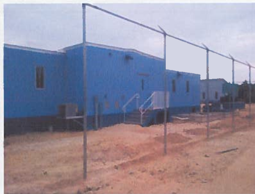
Security Fence installation in progress – Monday May 4
