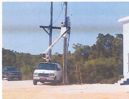
Security Camera installation in progress – Friday May 8
