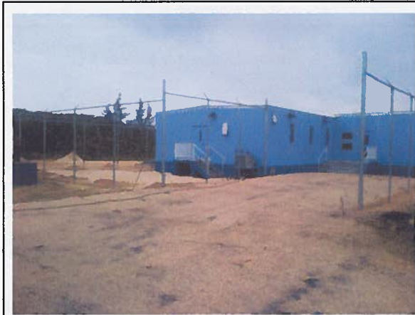
Security Fence installation in progress – Monday May 4
