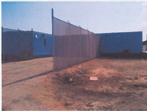
Security Fence installation in progress – Friday May 8
