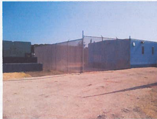
Security Fence installation in progress – Friday May 8
